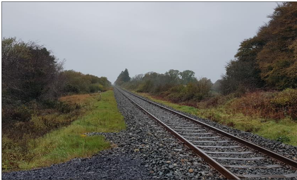
Figure 16. Survey Point 6 – View to Southeast
