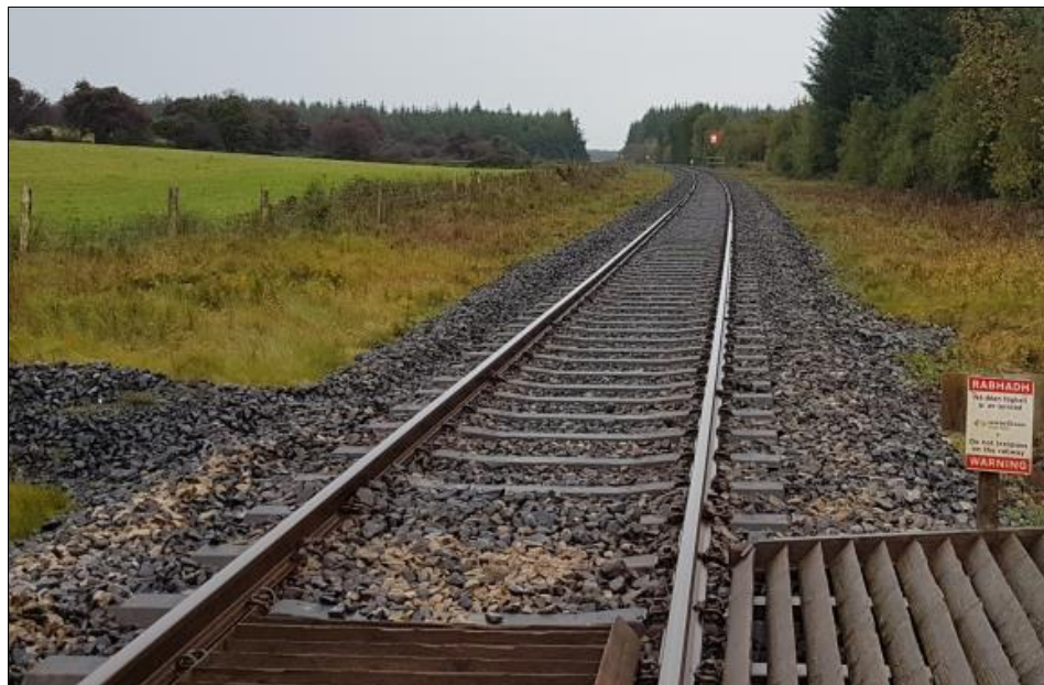
Figure 10. Survey Point 3 – View to Southeast
