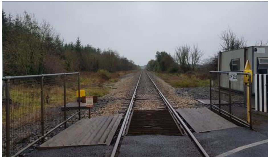
Figure 14. Survey Point 5 – View to Southeast
