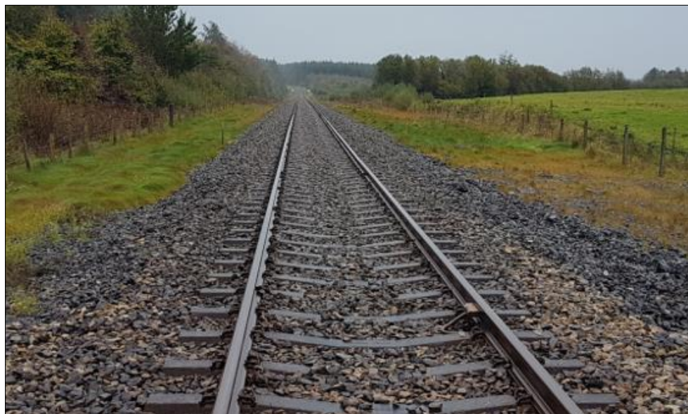
Figure 8. Survey Point 2 – View to Southeast
