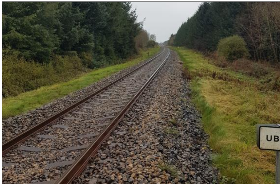
Figure 6. Survey Point 1 – View to Southeast
