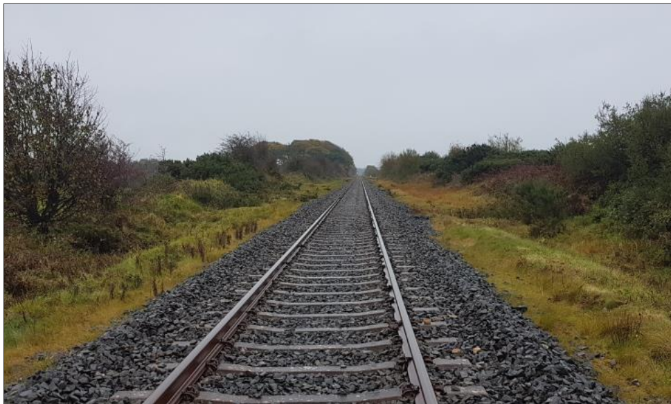
Figure 18. Survey Point 7 – View to Southeast
